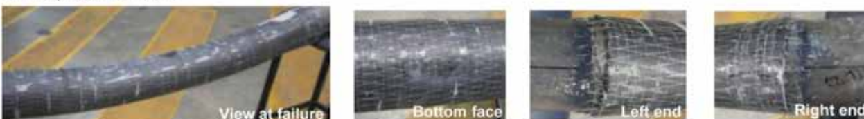
Figure 18. Failure mode of tested beams
