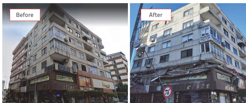
Figure 15. Previous and post-earthquake damage to a building in Iskenderun–Hatay
