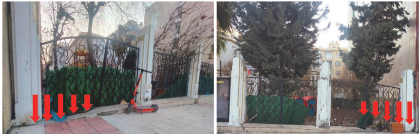
Figure 8. Liquefaction and sand slides observed in İskenderun–Hatay due to earthquake
