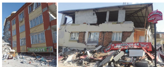
Figure 16. Soft-story buildings in Antakya–Hatay collapsed during the earthquake
