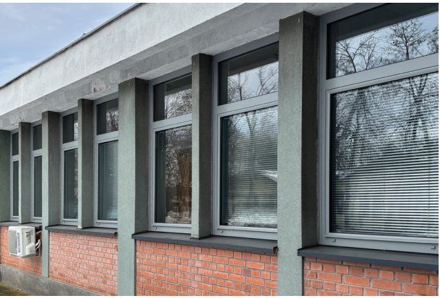
Figure 4. Case study: Office space window at the Faculty of Technology in Banja Luka
