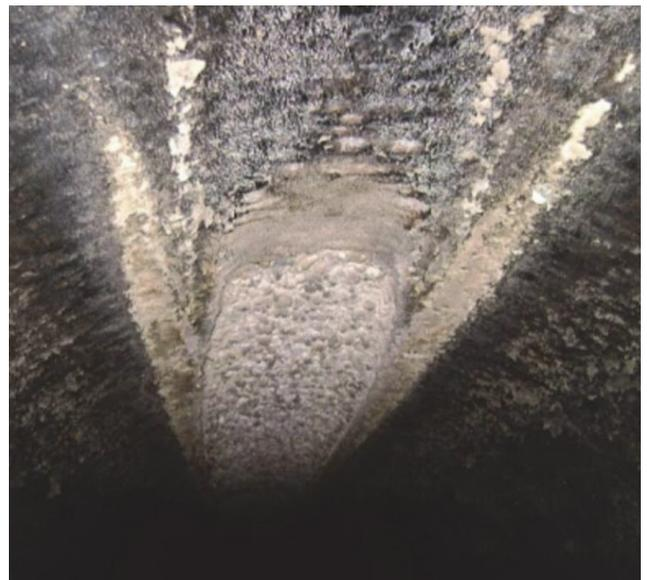
Figure 15. Surface corrosion and exposed aggregates [76]
