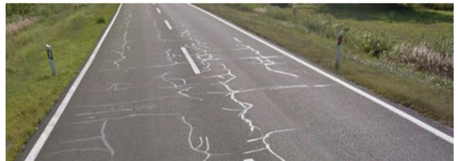
Figure 4. Temperature cracks on D28 Bjelovar bypass from km 7+000 to km 7+500
