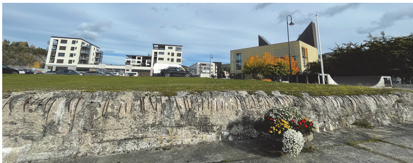
Figure 4 Remediated "brownfield" areas Nottodden in Norway [33]
