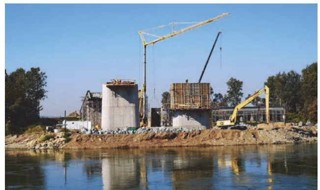
Figure 7. Construction of pier S4, Bosnia and Herzegovina side
