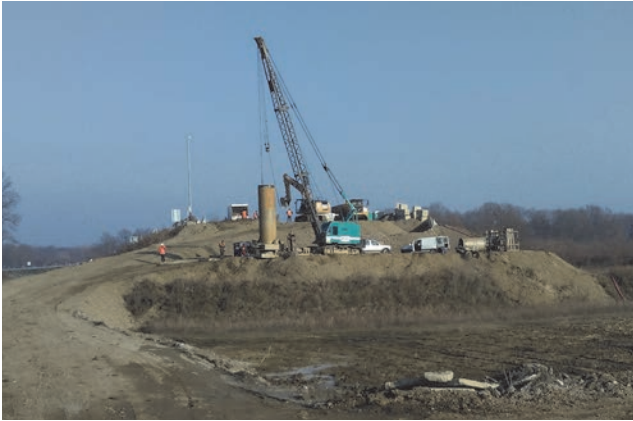
Figure 4. Pile drilling rig at abutment U1, Croatian side
