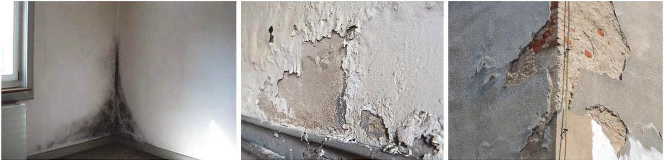
Figure 8. Damage to the envelope as a result of poor control of heat and moisture transfer
