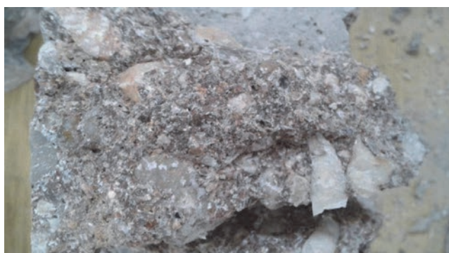
Figure 31. Seepage through concrete
