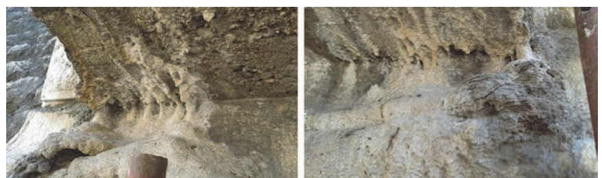
Figure 17. Deposits at left abutment - east side
