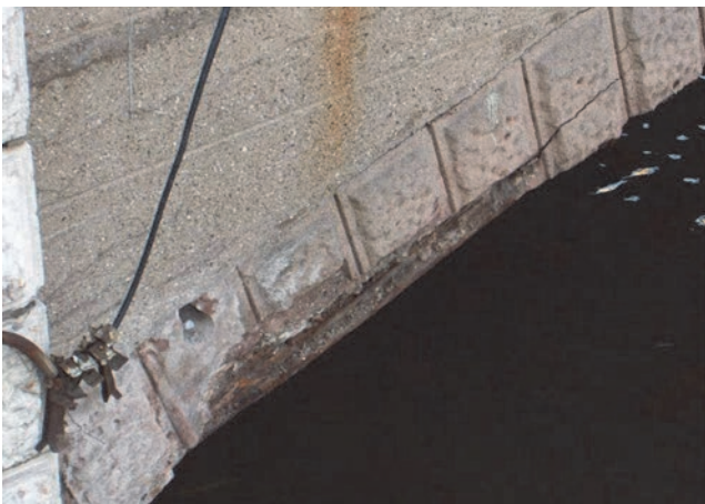
Figure 12. Horizontal cracks on the walls: east façade - upstream side
