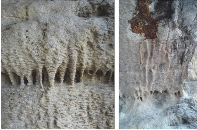
Figure 18. Deposits at left abutment - east side
