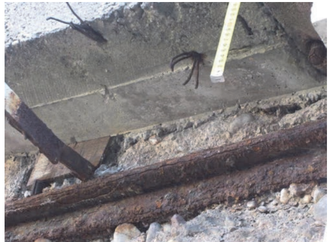
Figure 9. Corrosion of top rigid reinforcement - east façade-upstream side
