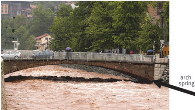
Figure 14. Flooding in May 2014
