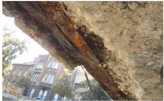
Figure 13. Corrosion of rigid reinforcement at bottom side of the arch - east façade - upstream
