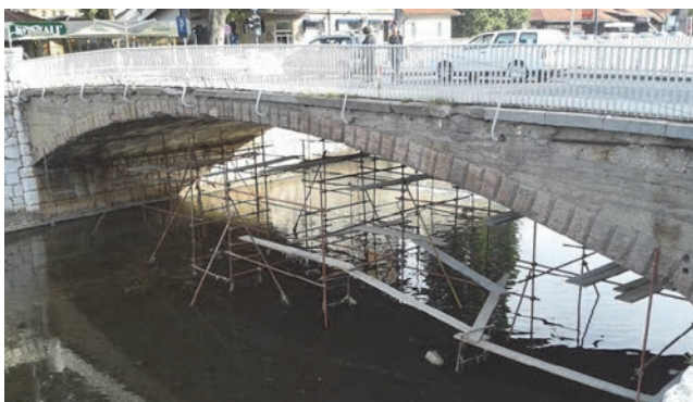
Figure 5. Careva Ćuprija Bridge with scaffolding during investigation works in 2015 [5]
