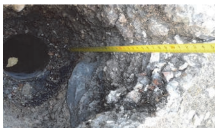
Figure 24. Waterproofing tar layer
