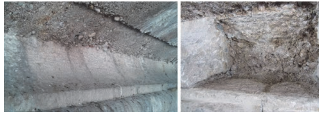
Figure 21. Abutment stone blocks at the left bank of the river and situation after their removal
