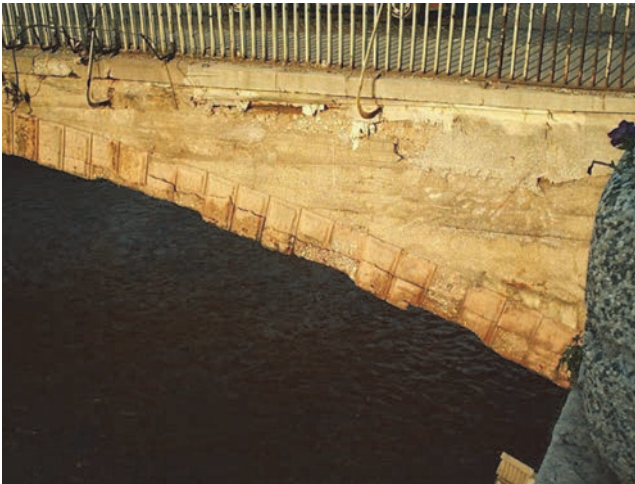
Figure 11. Detachment of decorative elements, horizontal cracks in concrete on the arch, and corrosion at the railing support - east façade - upstream side
